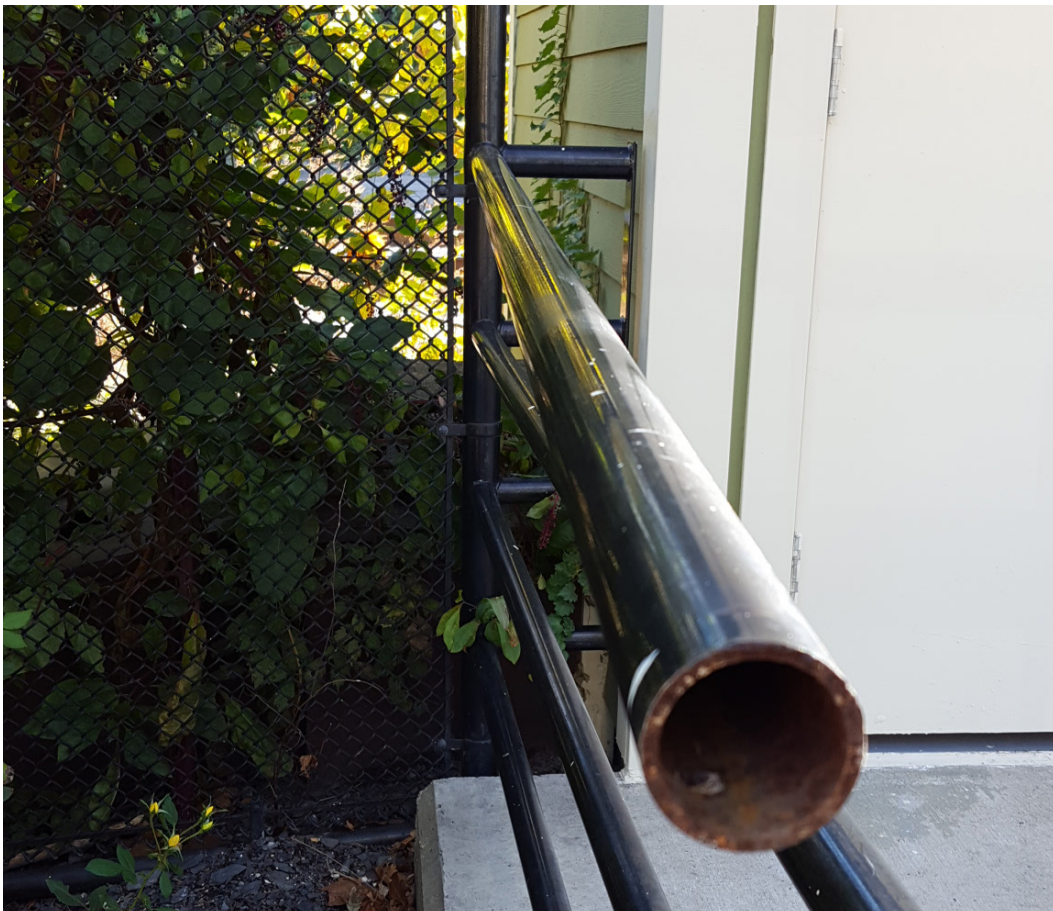
PHOTO #2 OF BROKEN RAILING AT COMPOSTING TOILETS
