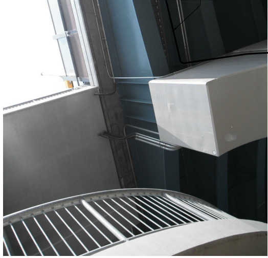
BRIDGE PIER MOUNT VERTICAL RISER
