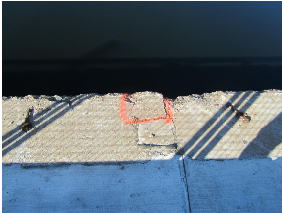
PHOTOS OF "TYPE 1" REPAIRS (ITEM SP-12A)
