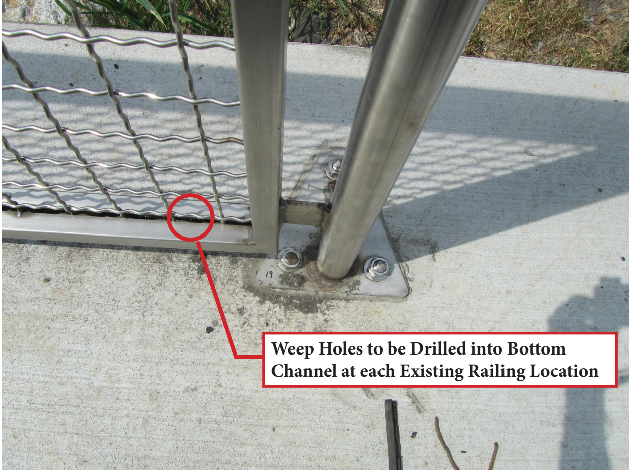
REPRESENTATIVE PHOTO FOR WEEP HOLE DRILLING (REFER TO EXHIBIT "E" UNDER SECTION 000150 FOR DETAIL)
