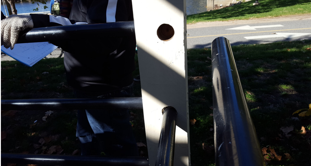
PHOTO #1 OF BROKEN RAILING AT COMPOSTING TOILETS
