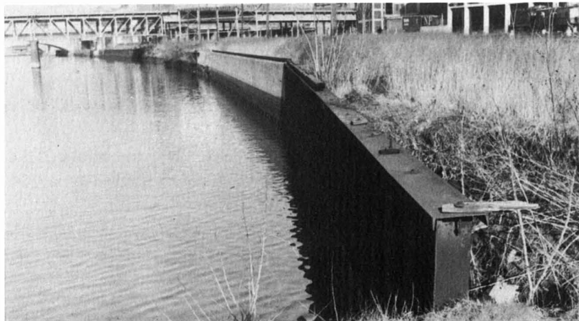
Bulkheads south of Walnut Street
