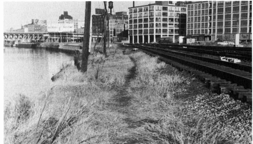
Limited space between tracks and the River
